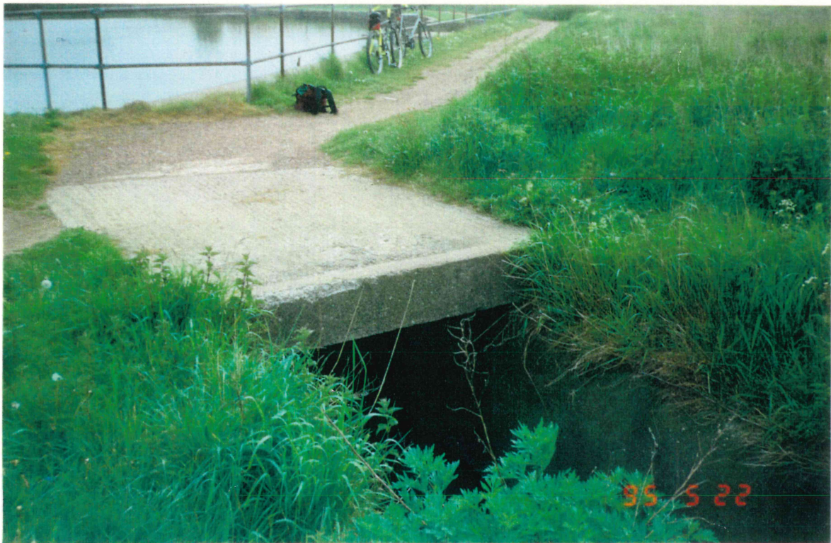
PHOTOGRAPH 2/13 - Concrete Slab Bridge
