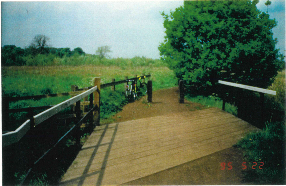
PHOTOGRAPH 3/22 - Timber Decking to Bridge
