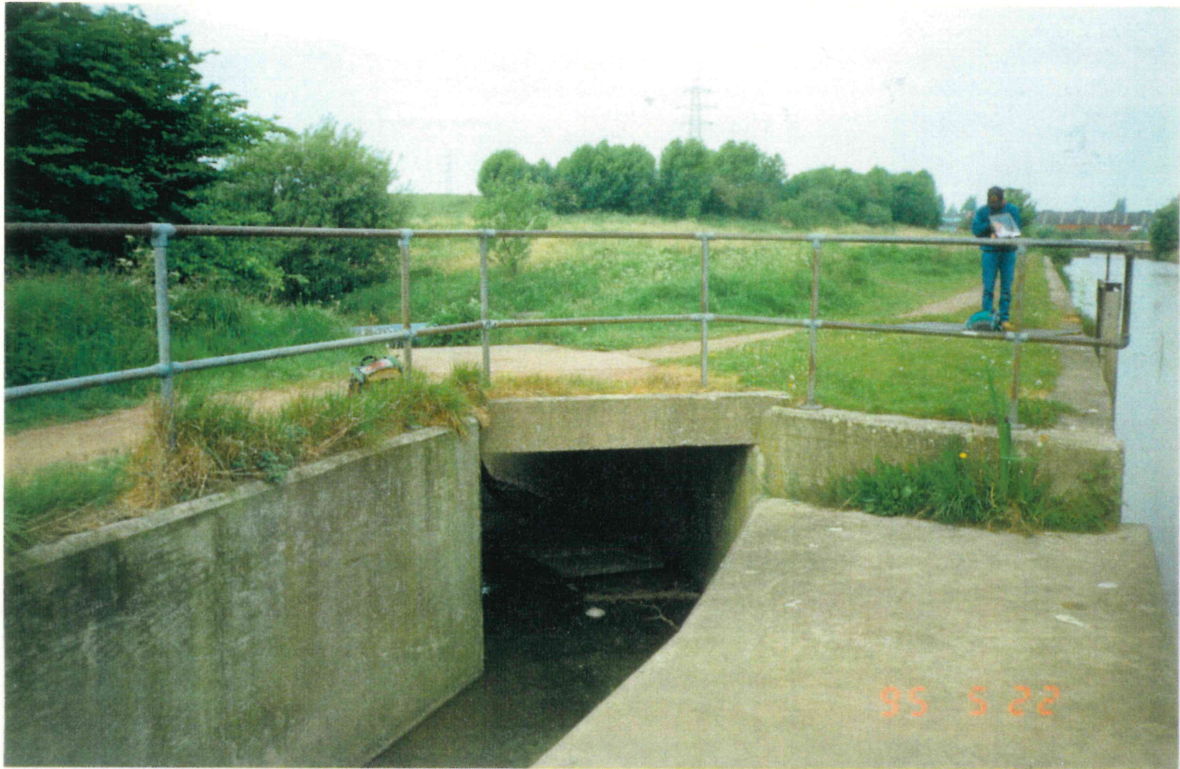
PHOTOGRAPH 2/12 - Concrete Channel Behind the Overflow Weir
